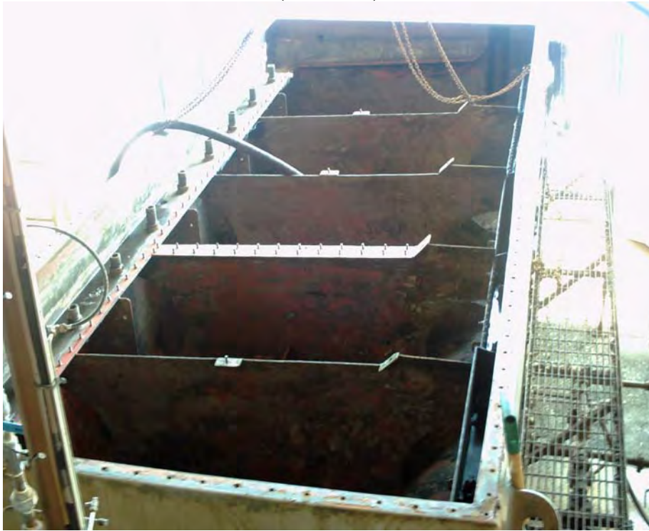
The photo shows the top cover plate removed and the IGF Cleaned by Enviro-Tech Systems Personnel
