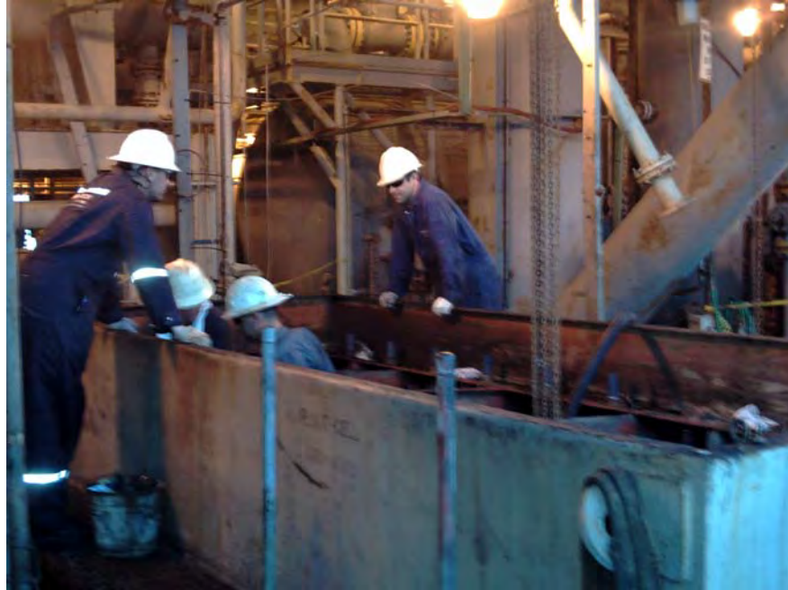
The photograph shows the Enviro-Tech team working to install new internal parts.
