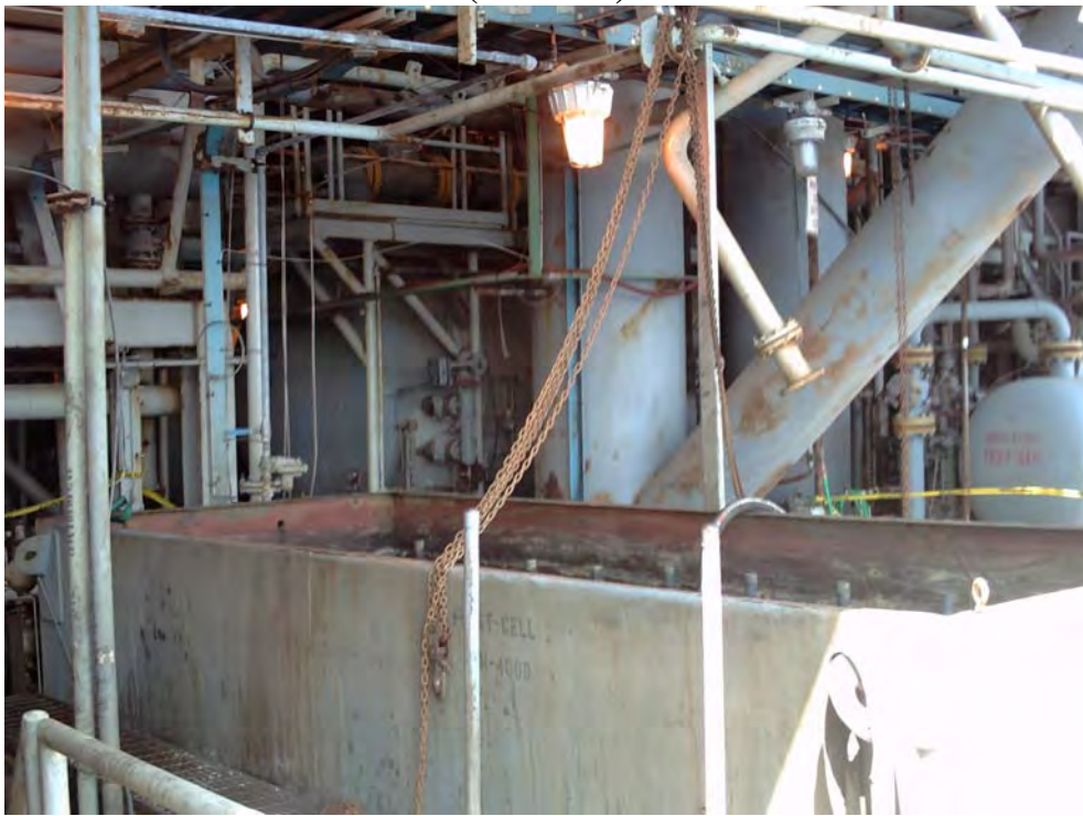
Starting to disassemble the existing IGF
