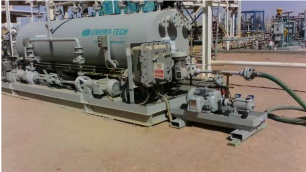
Figure 10. Field Installation of IGF + DGF Water Treatment Package
